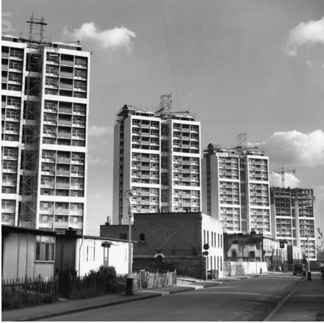
Prefabrication, Brandon Estate. Hulton Archive
