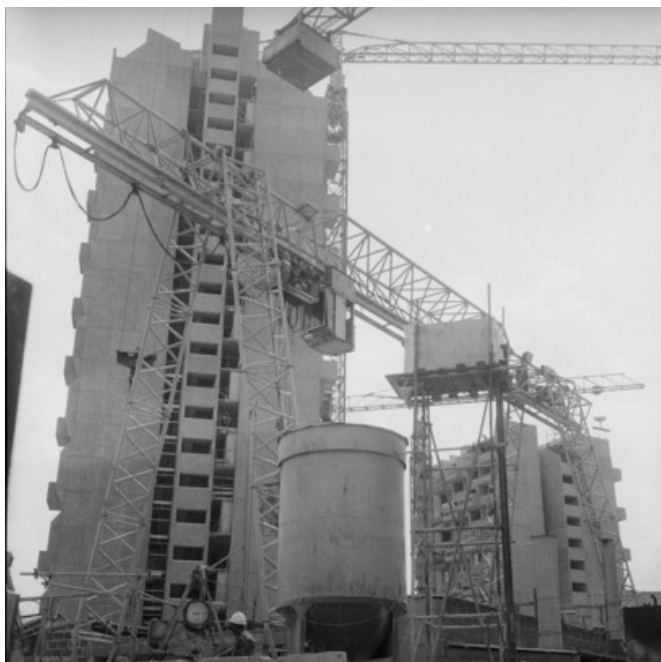
Lambeth estate under construction 1968. Museum of London
